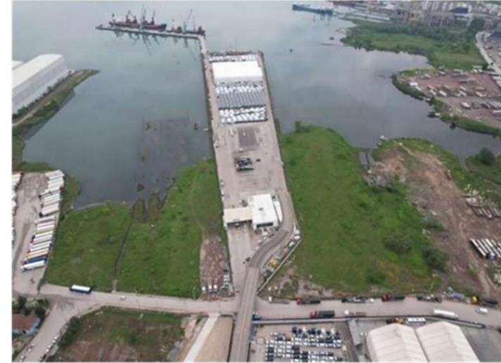
Photo 3: Forecourt Area and shoreland to be developed
