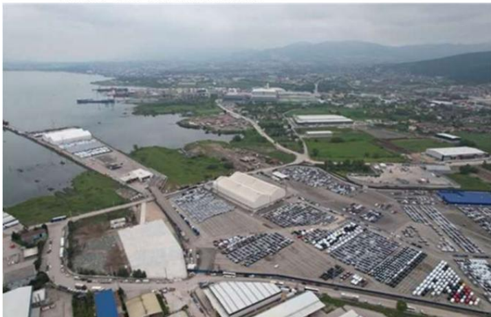
Photo 4: Autoport Facility as seen from the Landside
