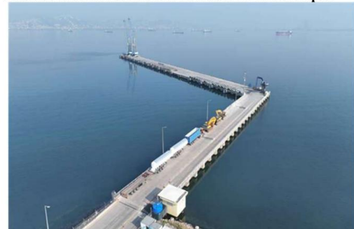
Photo 6: Existing Pier Area which will be developed
