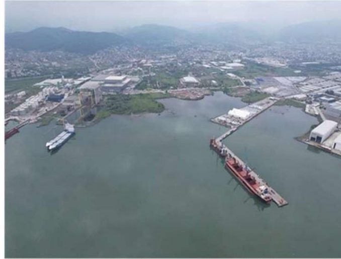
Photo 2: Autoport facility as seen from the Marmara Sea
